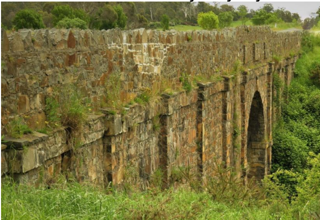
Kerry Lodge Bridge by Mark Brunken
