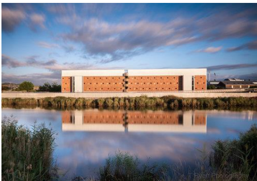
UTAS Accommodation Block on the North Esk River. Photo by Thomas Ryan.
