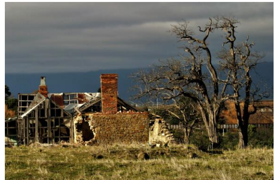
Abandoned house at Avoca (Mark Brunken)
