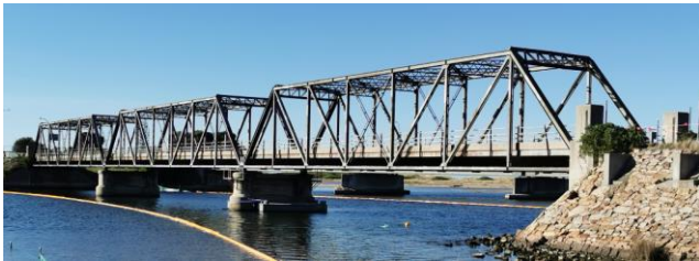
Old Scamander bridge now being demolished.
