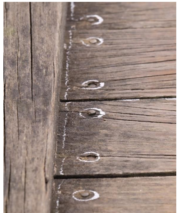
Rings of Ice around nail heads on the boardwalk at Tamar Island by Rod Oliver
