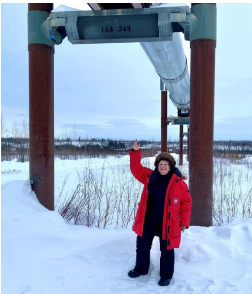
Part of the 800-mile oil pipeline from Prudhoe Bay to Valdez, Alaska.
